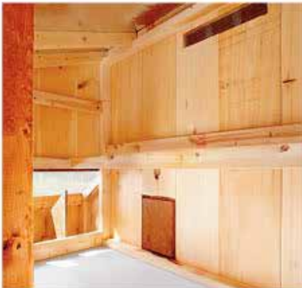
Interior view of L35 (page 71)
