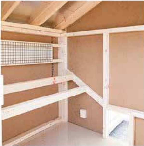
Interior View Of Roost, Ventilation Lid And Chicken Door- Q44, Q46, Q48 (pages 44-47)
